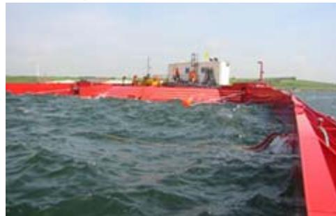
The Wave Dragon structure is stationary set up to face the predominant wave conditions. The turbines are the only moving parts.
