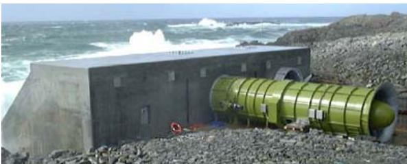
world's first commercial scale wave energy converter, located on the coast of Islay in the Highlands of Scotland. It is the smallest of Wavgen's shoreline energy modules, and generates 0.5MW of power for local communities. There are now plans for Wavgen to install a LIMPET style generator on the Faeroe Islands.
